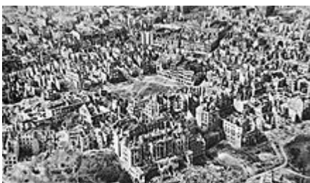
Warsaw destroyed , photo taken January 1945
